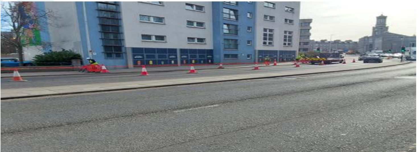
Phase 4 scaffolding lane closure and footpath restrictions.
